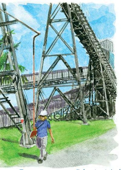
Terragen is a power producer that supplies electricity to the Central Electricity Board (CEB), as well as electricity and steam to Terra's sugar mill, through two 35 MW thermal units. Operating in a joint venture partnership with French company Albioma, we generate electricity and steam by burning bagasse and cane trash during the crop season (from July to December), and imported coal during the intercrop season.
